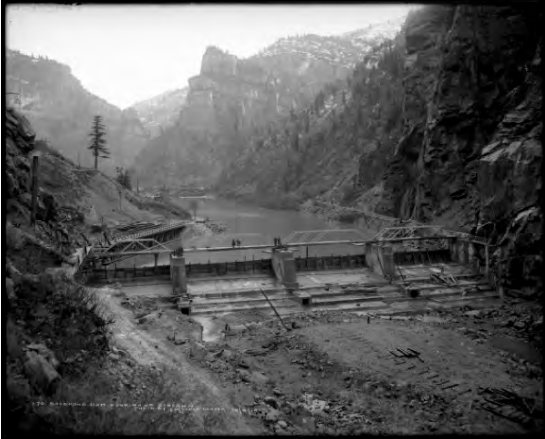
Illustration A 4.10: The Shoshone Dam, on the Colorado River several miles above the powerhouse, was an engineering achievement. Steel gates known as bear traps could be raised or lowered, depending on river flow, to ensure diversion into the powerplant's intake tunnel in the cliff at the left side. Charles McClure captured the upstream view in 1910. Courtesy of Denver Public Library, MCC-3850.
