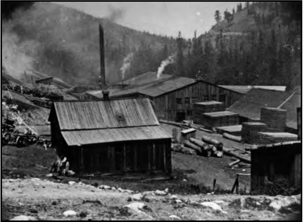
Illustration B 2.2: The I-70 corridor featured a few large sawmills comparable to the W.H. Woods plant in Winter Park, photographed around 1910. The large building in center background houses the saw-blades, steam engine, boiler, and planing machinery. A residential cabin stands in the foreground, raw logs are stacked in rows in the distant background, while finished lumber is stacked at right. Courtesy of Denver Public Library, X-14066.
