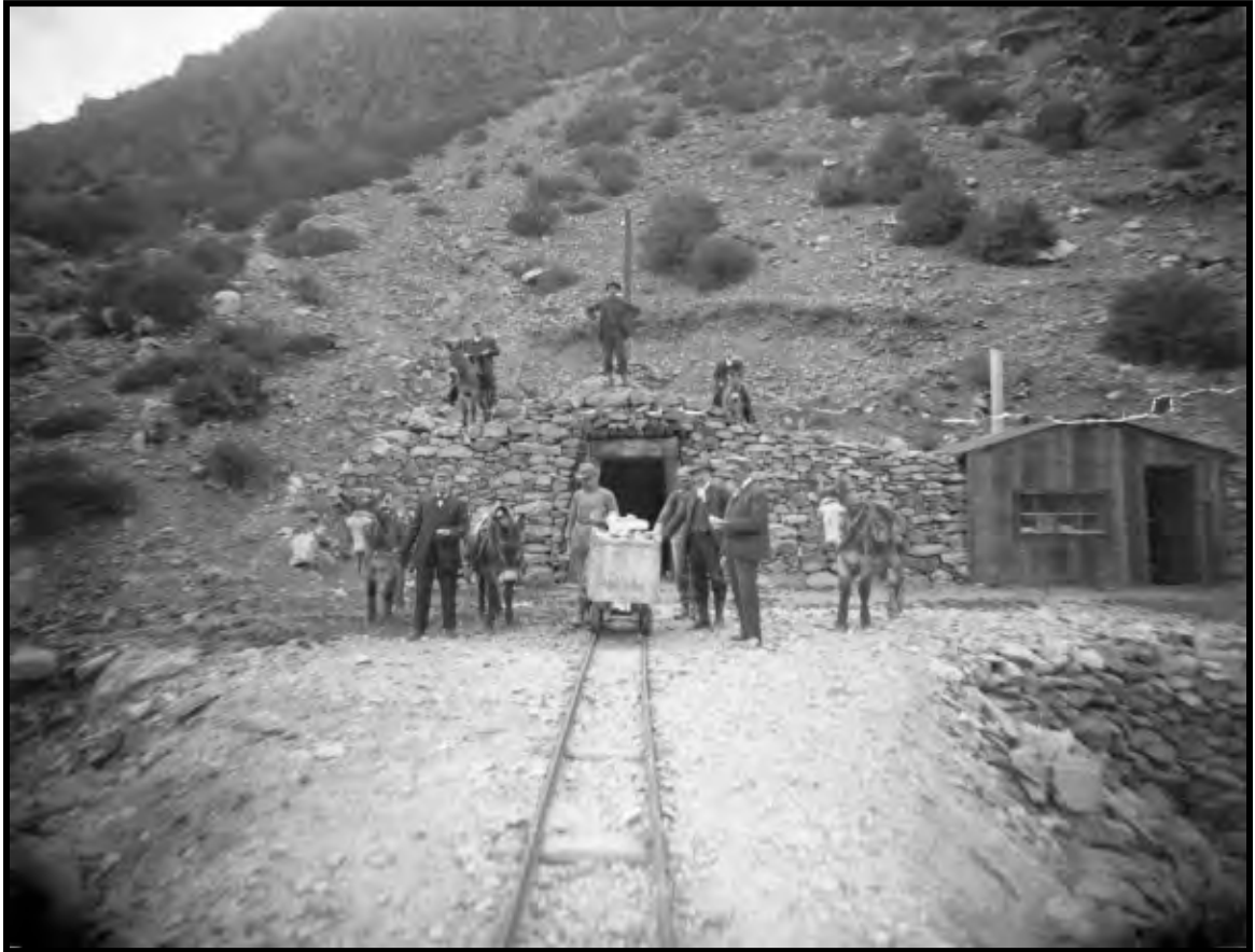
Illustration B 1.7: Most tunnel mines, such as this operation near Georgetown during the 1890s, were small and simple. Surface facilities consisted of a blacksmith shop, tunnel portal, rail line, ore bin, and little else. Even when buildings and structures are gone, tunnel mines may be eligible for the NRHP if the archaeological features and artifacts clearly represent the operation. Courtesy of Denver Public Library, X-61651.
