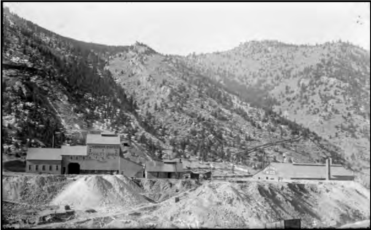
Illustration A 1.2.22: The Stanley Mine was a result of the mid-1890s gold boom in eastern Clear Creek drainage. The operation, a consolidation of properties on both sides of the valley, became one of the most advanced mines in the region. The building at left is an icon visible from I-70 today. Harry H. Buckwalter photographed the southwest view around 1900. Courtesy of Denver Public Library, CHS-B1486.
