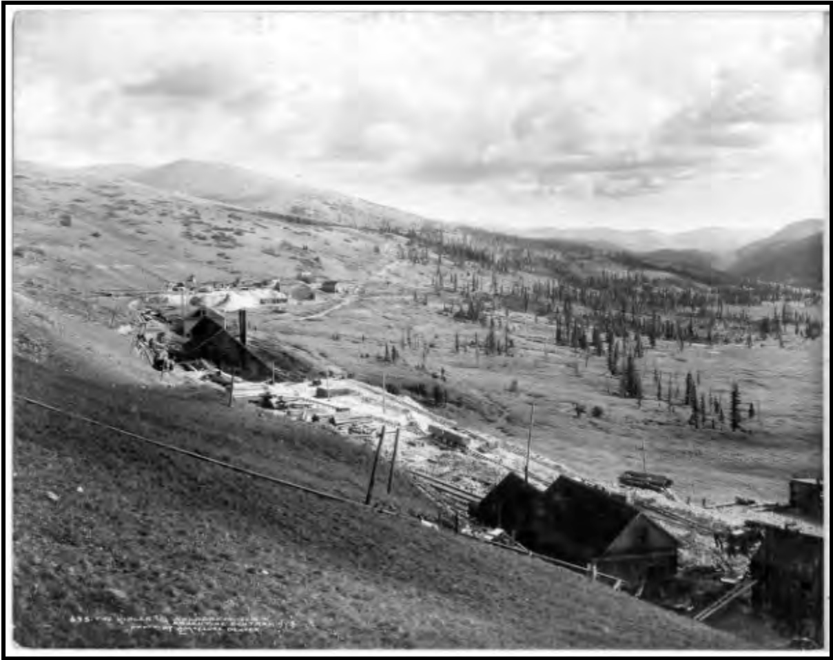
Illustration A 1.2.26: In the northeast overview, the Vidler Tunnel complex is in the foreground and Wilcox Tunnel and settlement of Waldorf is in the left background. Both were important operations in the Argentine Mining District from 1907 through 1910. Waldorf was center of Edward Wilcox's mining empire, including the Wilcox Tunnel and mill, Argentine Central Railroad terminus, and a tourist hotel. The abandoned townsite of Argentine was on the valley floor at far right, and Georgetown lay over the ridge beyond. Charles McClure took this north view around 1910. Courtesy of Denver Public Library, MCC-695.
