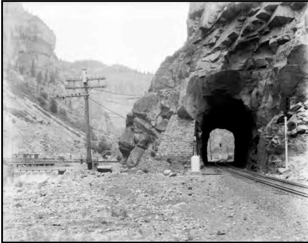
Illustration B 5.2: This circa 1925 George L. Beam photo shows a typical railroad tunnel and right-of-way objects and structures in Glenwood Canyon by the Shoshone diversion dam, left background. The utility pole is a structure, and the signal lights at right objects. All are contributing elements of the railroad as a resource. Courtesy of Denver Public Library, GB-6399.
