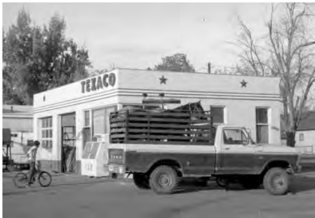
Illustration B 8.24: Texaco Oblong Box filling station, Ignacio, Colorado. Courtesy Denver Public Library, X-17788, ca. 1980-1990
