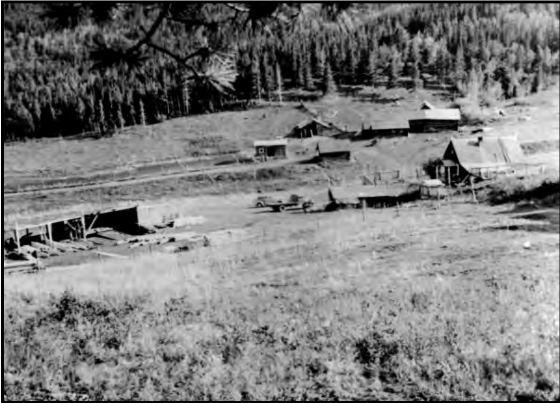
Illustration B 2.1: Most of the sawmills in the I-70 corridor were small facilities such as this one photographed near Silver Plume in 1938. They were simple for portability and relocation to fresh forests. The sawmill, frame enclosing the saw-frame, and building surrounding the saw-blades and engine are at left. Finished lumber and logs are stockpiled near center, and workers' housing is right. Courtesy of Denver Public Library, X-17668.
