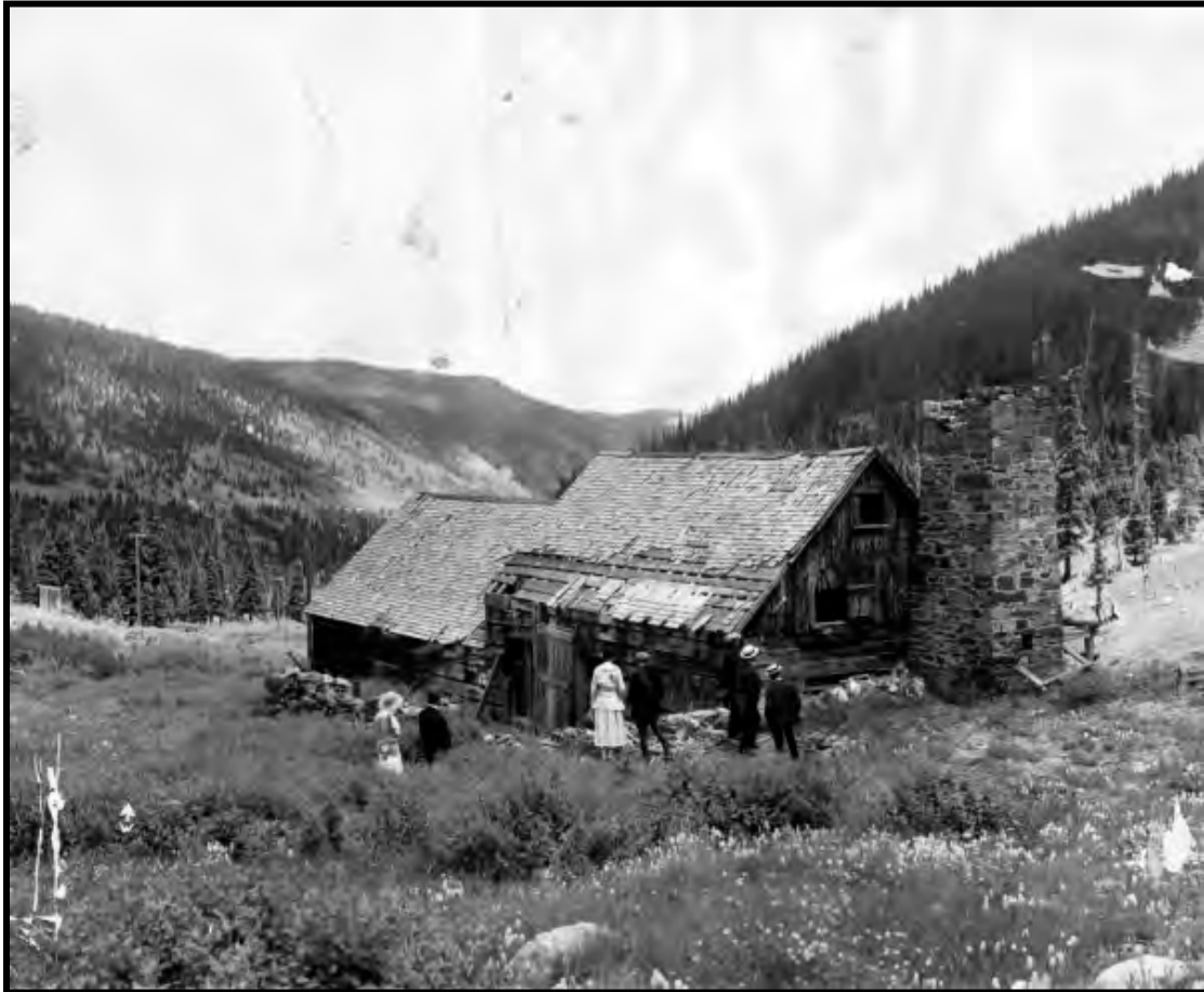
Illustration B 1.15: When the Dibben Smelter at Argentine was photographed during the late 1890s, it had already been long abandoned. The facility is typical of the smelters built in Clear Creek drainage during the late 1860s and early 1870s, with local stone chimney and furnace, and small building built over several stairstep foundations. Masonry and foundations are all that remain from most smelters of the vintage. Courtesy of Denver Public Library, X-61397.
