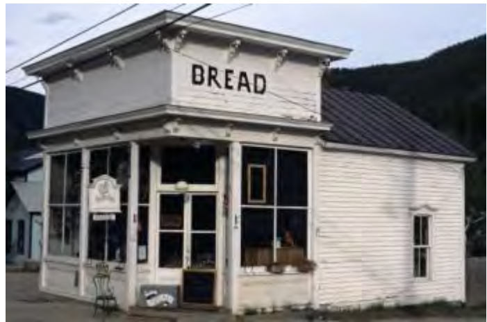
Illustration B 8.-18: Sopp and Truscott Bakery, Corner Commercial building, Silver Plume, Courtesy of Denver Public Library, AUR-962, 2010
