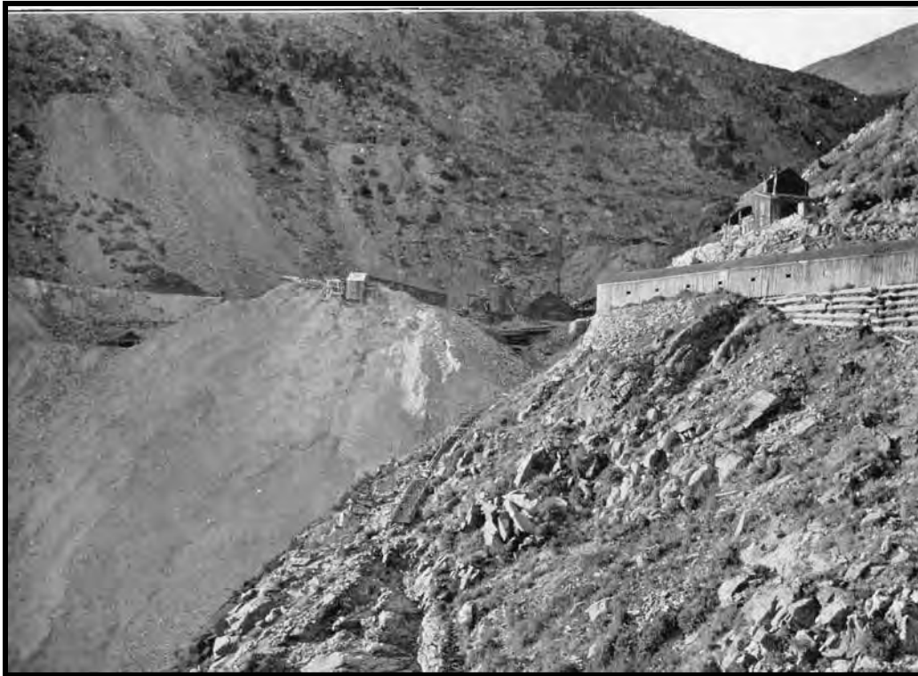
Illustration A 1.2.12: The Seven-Thirty Mine was typical of Silver Plume's numerous silver producers. The mine was a tunnel operation with massive waste rock dump piled on a steep mountainside. Several times, these dumps gave way and cascaded onto buildings in town below. When this northwest view was taken during the 1890s, little had changed. Source: Spurr, 1908.
