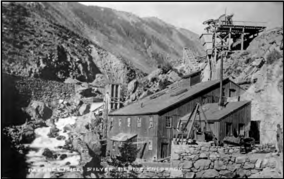
Illustration B 1.13: The Pay Rock Mill, on the north side of Clear Creek near Silver Plume in 1880, is a good example of a typical concentration facility. The building descends over a series of stairstep foundations, which are often all that remain at mill sites today. Courtesy of Denver Public Library, X-61593.
