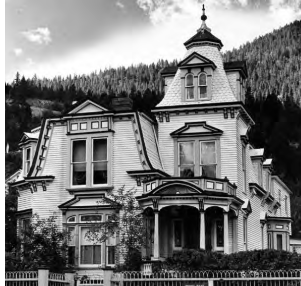
Illustration B 8.5: Maxwell House, Second Empire style dwelling, Georgetown. Courtesy Denver Public Library, X-1277, ca. 1970.
