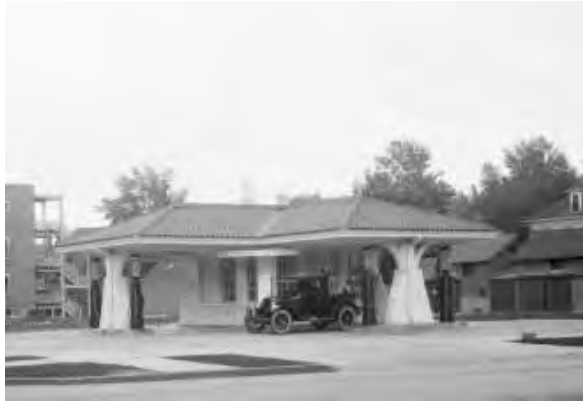
Illustration B 8.21: House with Canopy filling station, Denver, Colorado. Courtesy of Denver Public Library, X-23806, ca. 1920-1930.
