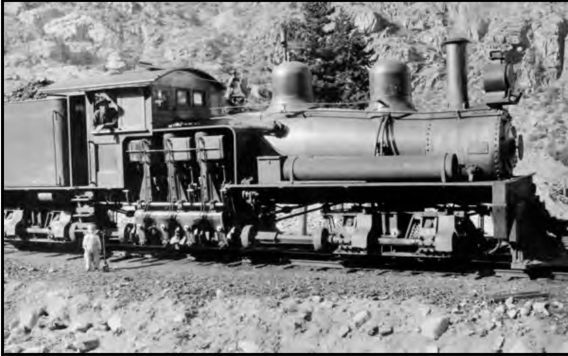
Illustration A 5.8: This side-gear locomotive, known as a Shay design, made the Argentine Central Railroad possible. The Shay was the only type capable of pulling cars up the tortuous and steep grades from Silver Plume into the Argentine Mining District. The photo was taken on the Argentine Central around 1910. Courtesy of Denver Public Library, X-17687.
