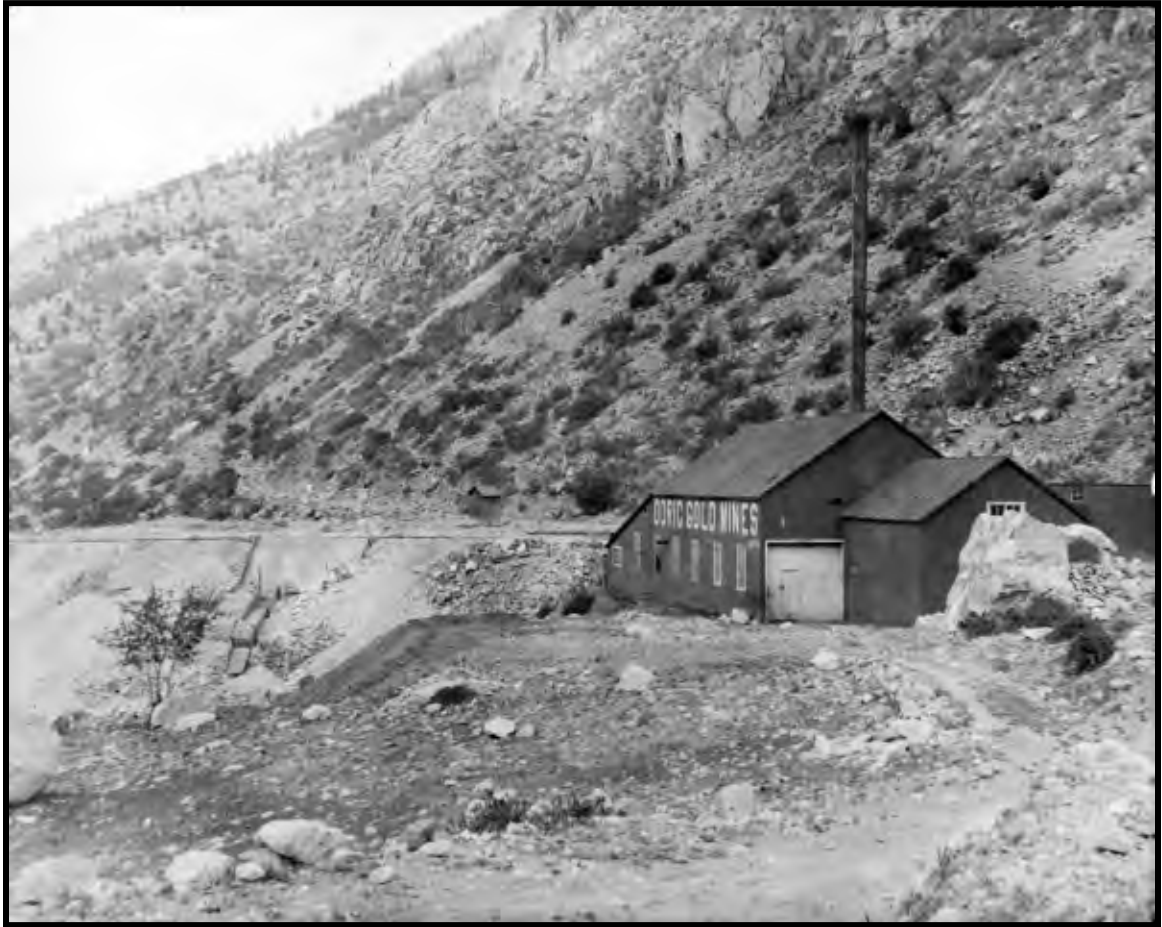
Illustration B 1.8: The Doric Mine near Georgetown, pictured around 1890, is typical of mechanized tunnel mines. A tunnel house encloses the tunnel portal, shops, air compressor, and steam boiler. A chute and decayed bin for ore lie on the waste rock dump's flank. Courtesy of Denver Public Library, X-61652.
