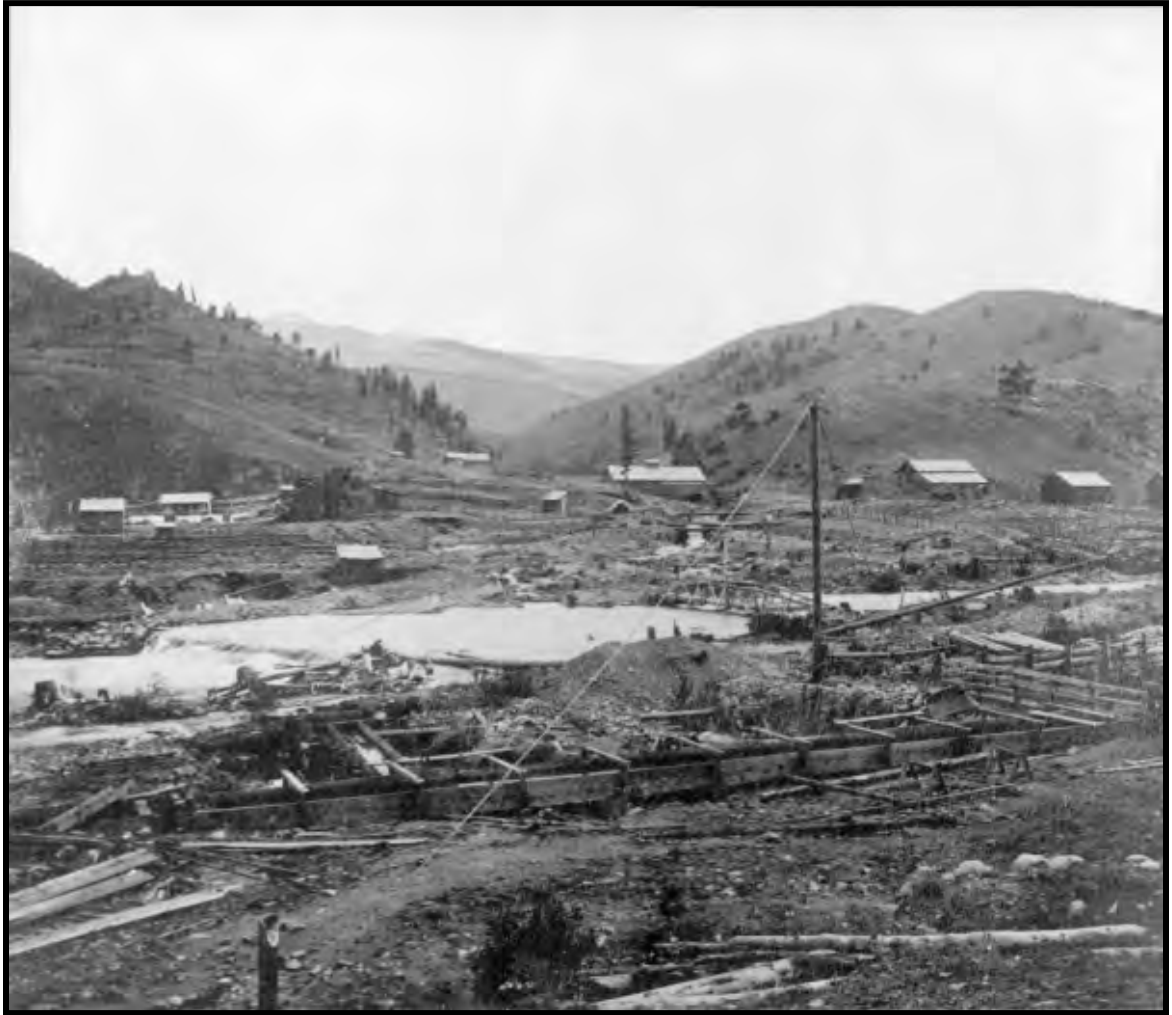
Illustration B 1.2: The 1867 photo captures a typical stream placer on Chicago Creek near Idaho Springs. The mine is characteristic of company operations with engineered sluices, log cribbing walls that retain pits, a hoisting derrick to remove boulders, and large tailings piles. Courtesy of Denver Public Library, X7604.
