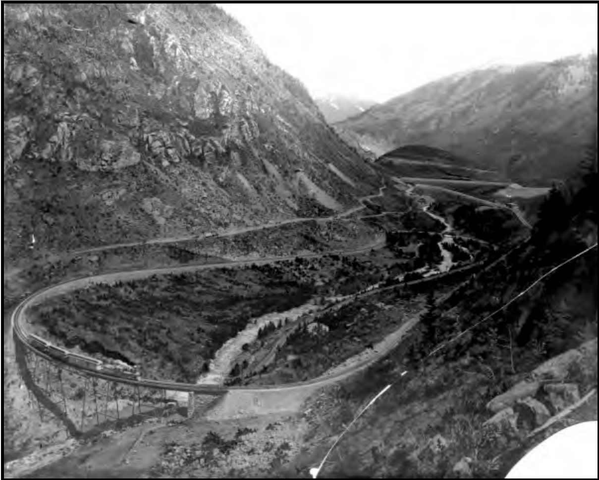
Illustration A 5.6: The sinuous series of curves and crossover on the Georgetown, Breckenridge & Leadville Railroad were collectively known as the Georgetown Loop. The crossover, made possible by the steel High Bridge, was an engineering feat recognized industry-wide. Enhanced by an impressive alpine setting captured in this 1880s William Henry Jackson photo, the Loop drew tourists from across the nation. Courtesy of Denver Public Library, CHS.J2201.
