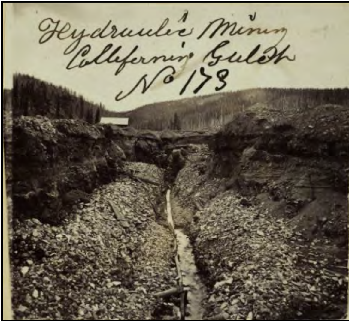
Illustration B 1.3: In hydraulic placer mines, the workings usually feature high and precipitous cut-banks, collections of boulders, and a central drain that directed effluent into sluices. The hydraulic monitor, water system, and sluices are out of view. Although the photo is in California Gulch near Leadville, hydraulic placers existed near Idaho Springs and Empire. Courtesy of Denver Public Library, X-19197.
