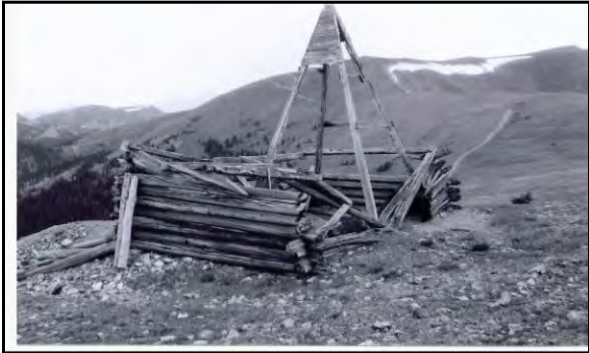
Illustration B 1.5: The Thompson Mine near Breckenridge in 2003, is characteristic of deep prospect shafts. These operations typically had a simple headframe and blacksmith shop enclosed in a shaft house. Additional property development is absent, and the waste rock dump limited in volume. Archaeological features represent the buildings and structures at most sites. Source: Eric Twitty.
