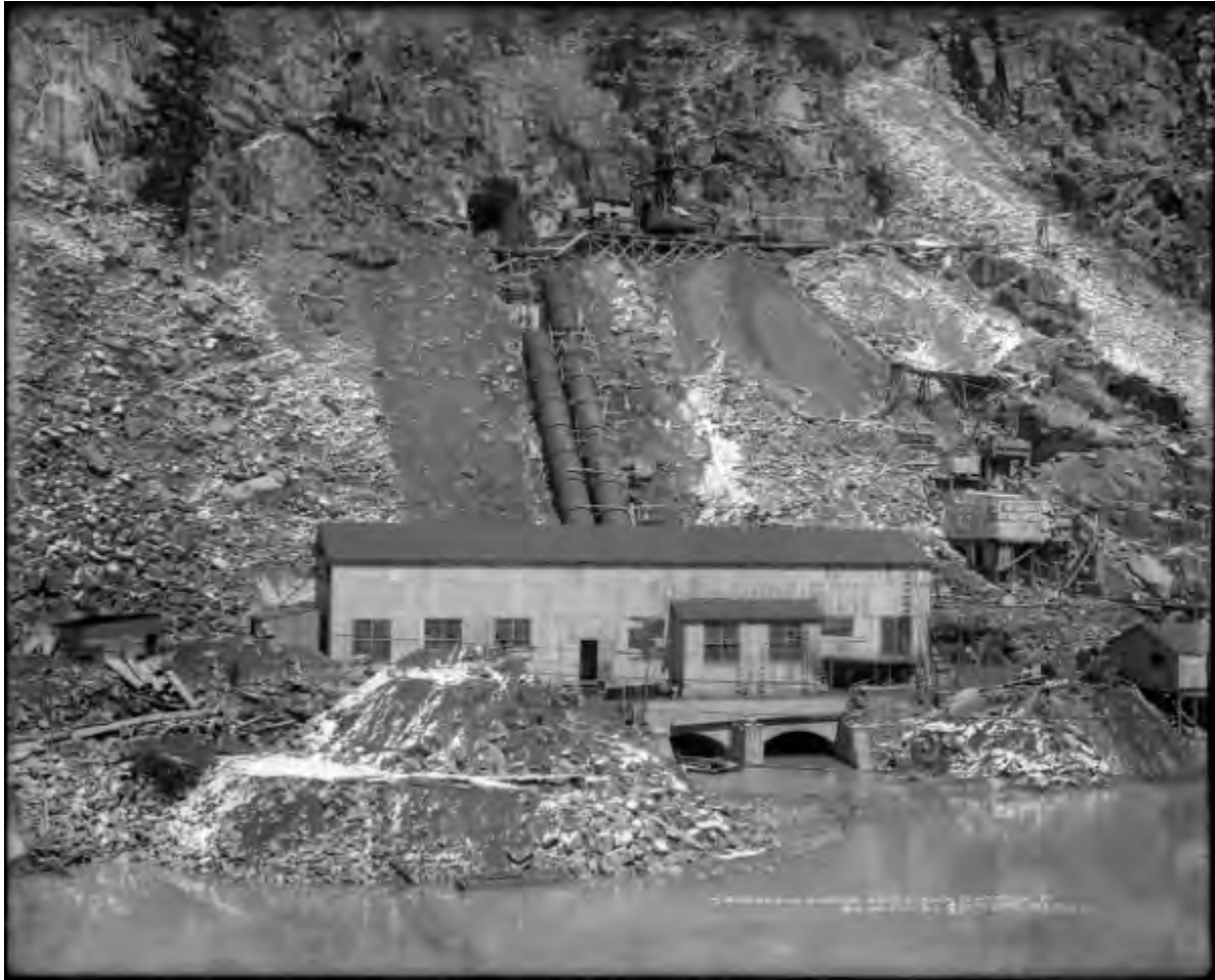
Illustration A 4.11: The Shoshone powerhouse, under construction in this Charles McClure 1908 photo, became the western terminus of a grid linking most of the principal towns in the central mountains. Water diverted from a dam upriver flowed through the tunnel in the cliff above, down through the penstocks, and into the building. Although modified, the system is still in operation today. Courtesy of Denver Public Library, MCC-3397.
