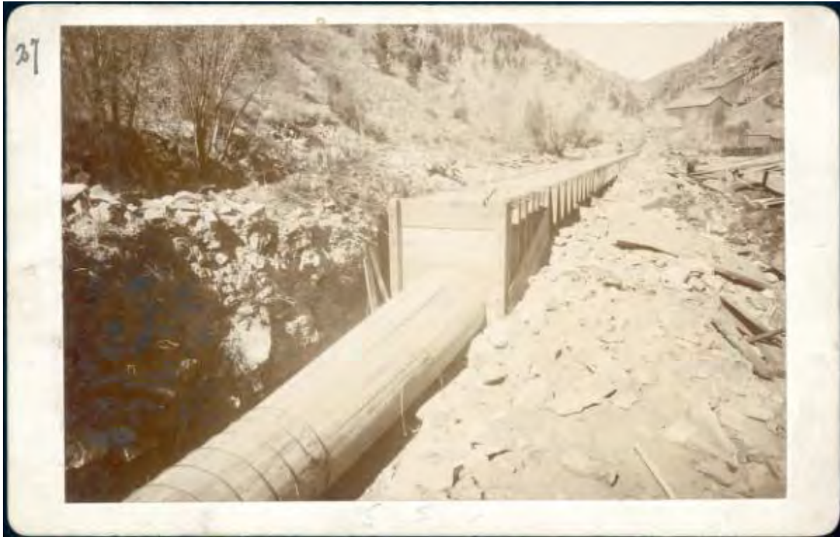
Illustration B 4.4: Infrastructure components include facilities and constructs in support of powerplants and their electric grids. Flumes and pipelines for hydropower, such as these in construction for the Stanley Mine near Idaho Springs in 1894, are the most common. Many have been dismantled and are now represented by archaeological features. Lachlan McLean took the photo. Courtesy of Denver Public Library, Z-4767.
