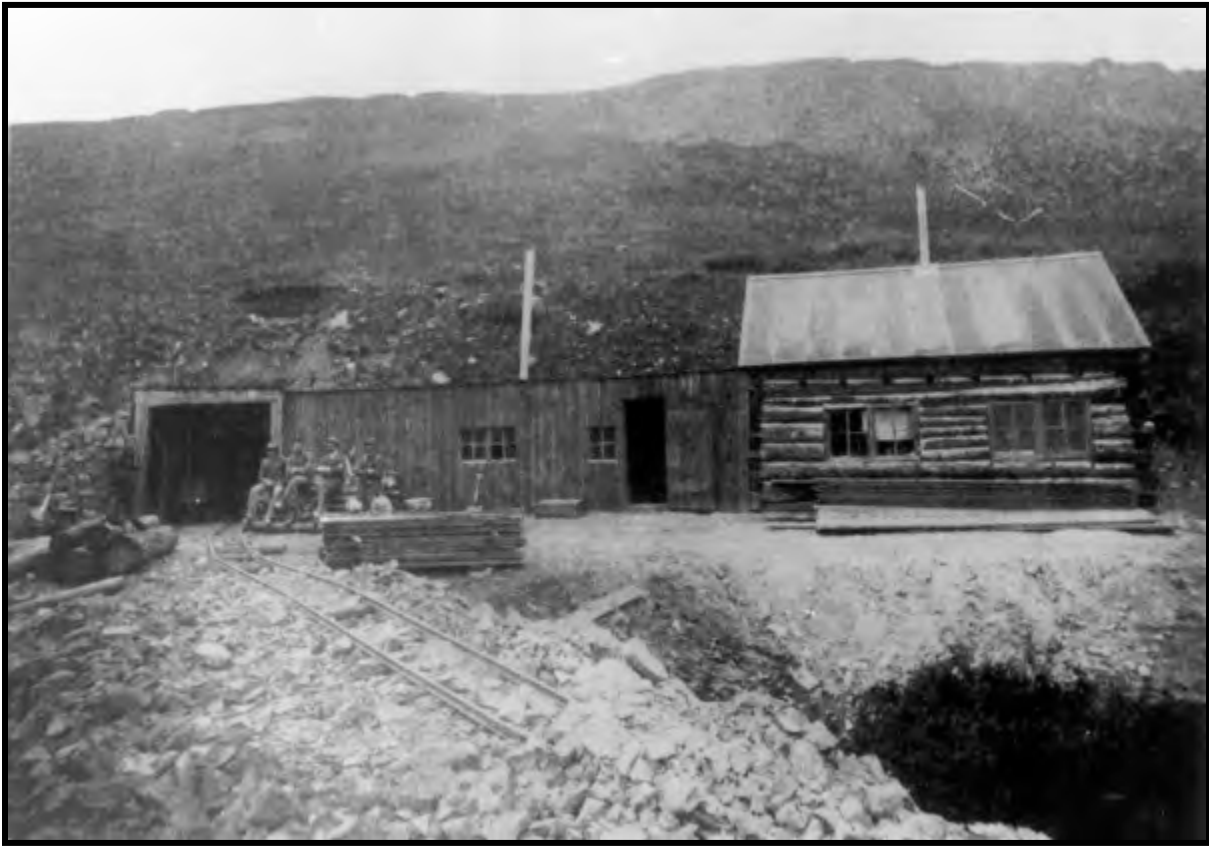
Illustration A 1.4.41: The buildings at the Vidler Tunnel, Argentine Mining District around 1905, are typical architecture at most mines. They were small and rough even when new, and not designed or constructed by professionals. Instead, miners planned them on-site to meet immediate needs, invested little capital, and used available materials. The building at left is a shed-type tunnel house with timber shop, and the log cabin at right may have been a blacksmith shop. The mine lacked machinery. Courtesy of Denver Public Library, X-61712.
