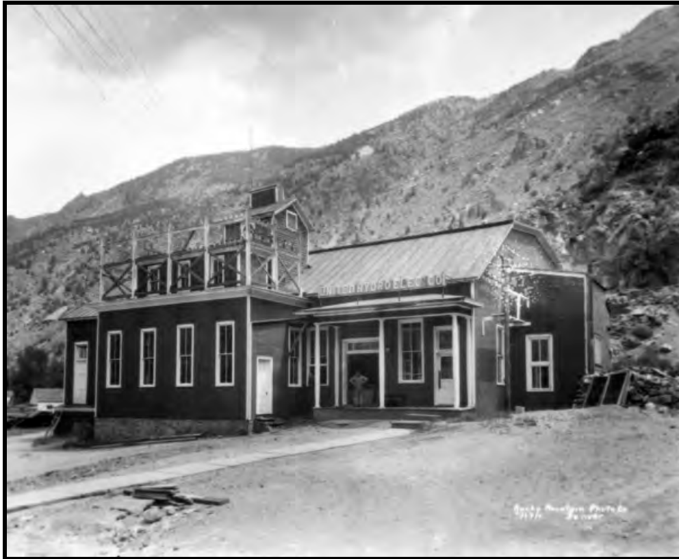
Illustration A 4.4: In 1900, United Light & Power built this Alternating Current hydro-plant in Georgetown as part of an expansion campaign to reach more mines in western Clear Creek drainage. The plant, among several others operated by the company, still functions. Courtesy of Denver Public Library, X-1029.
