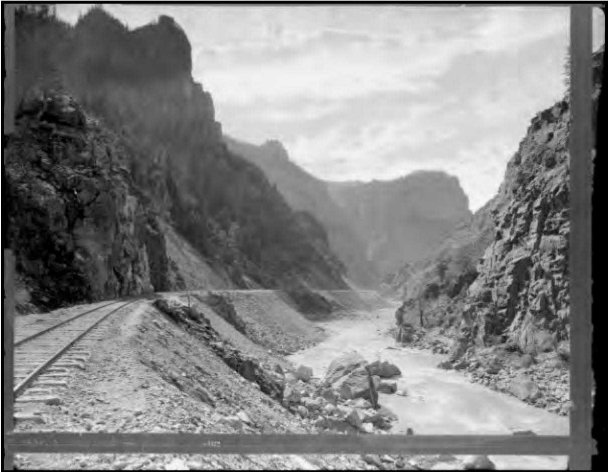
Illustration B 5.1: The late 1880s William Henry Jackson photo of the Denver & Rio Grande line through Glenwood Canyon exemplifies a typical railroad grade and common characteristics. Evident are cuts and fills to level the grade, and gentle curves and straight lines required by locomotives. The track consists of rails, ties, and a veneer of ballast over the carefully flattened surface of the gravel bed. Courtesy of Denver Public Library, CHS.J3885.
