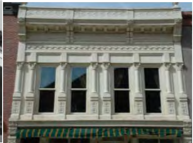
Illustration B 8.17: Mahr Building, Telluride, Colorado, with 1892 Mesker Bros. cast iron facade. Source: Carl McWilliams, 2007.
