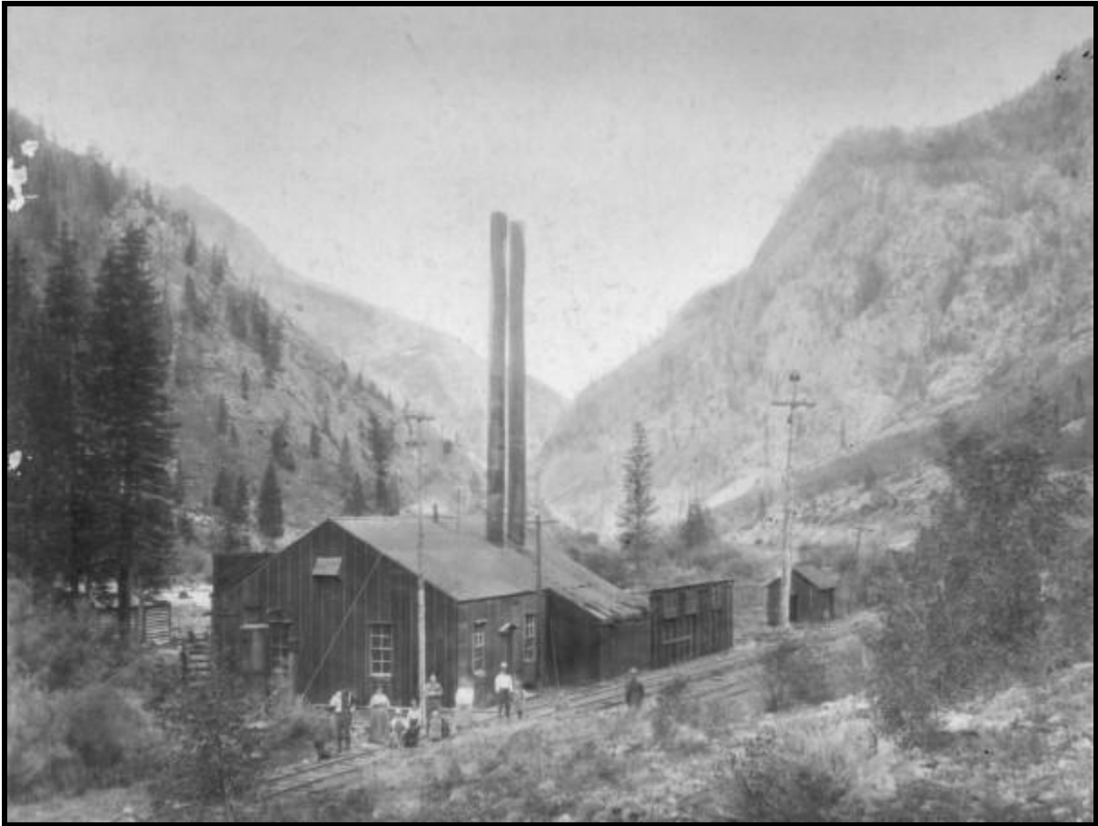
Illustration A 4.7: In the first decade of the twentieth century, the Dillon and Frisco area lacked a coordinated grid. Instead, several mining companies built their own powerhouses to provide electricity for themselves and associated communities. The Mary Verna Powerhouse generated for the Mary Verna and North American mines, and the settlement of Curtin. The powerhouse in this circa 1910 photo by Otto Westerman is a typical steam plant of the era. Courtesy of Denver Public Library, X-62730.
