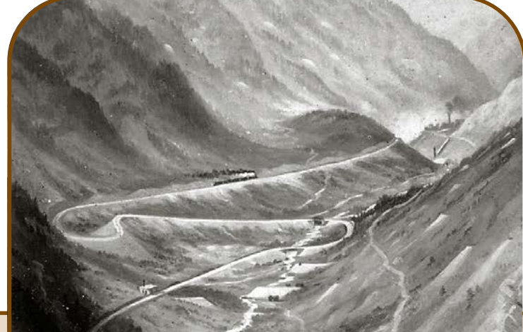
The Georgetown Loop, the famous narrow-gauge tracks of the Colorado & Southern Railroad. View looking upvalley toward the town of Silver Plume in the upper right. Because of its maximum grade up Clear Creek in a direct line from Georgetown to Silver Plume, this was the steepest 1875 percent grade for trains in the United States. This grade did not exceed 3 percent. This required 4.5 miles of railroad track that gully climbed Clear Creek valley, whereas, by direct line the distance is a little over a mile. From an 1890 painting by W.H. Jackson, (Temp 16).
