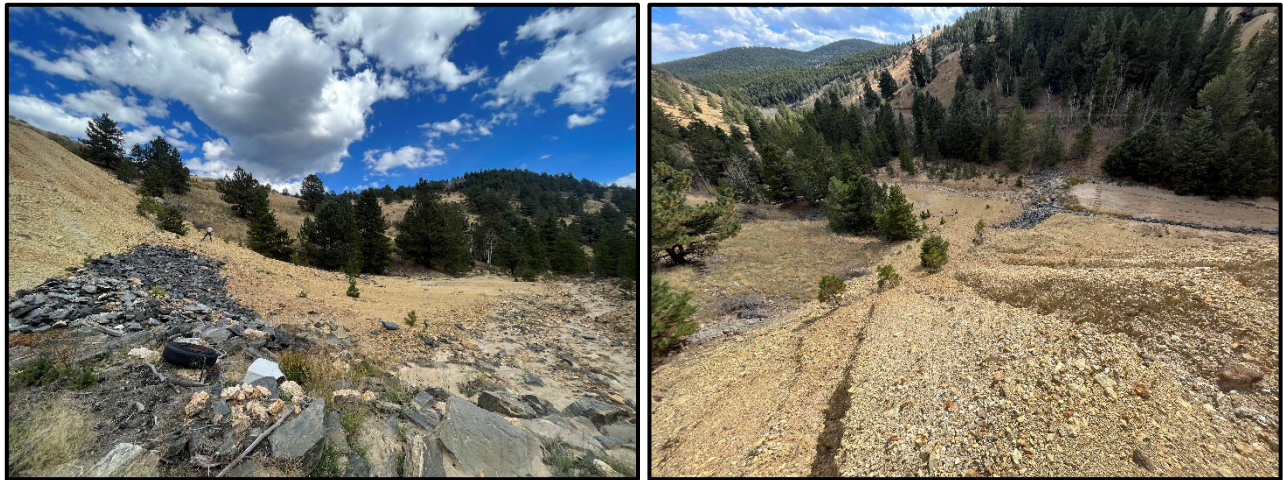
Figure 26. Site #158 – The base of the southeast portion of the waste pile where sediment flows directly into Russell Gulch (left) and the origination point of that sediment from the top of the waste pile where there’s significant gully erosion (right).
