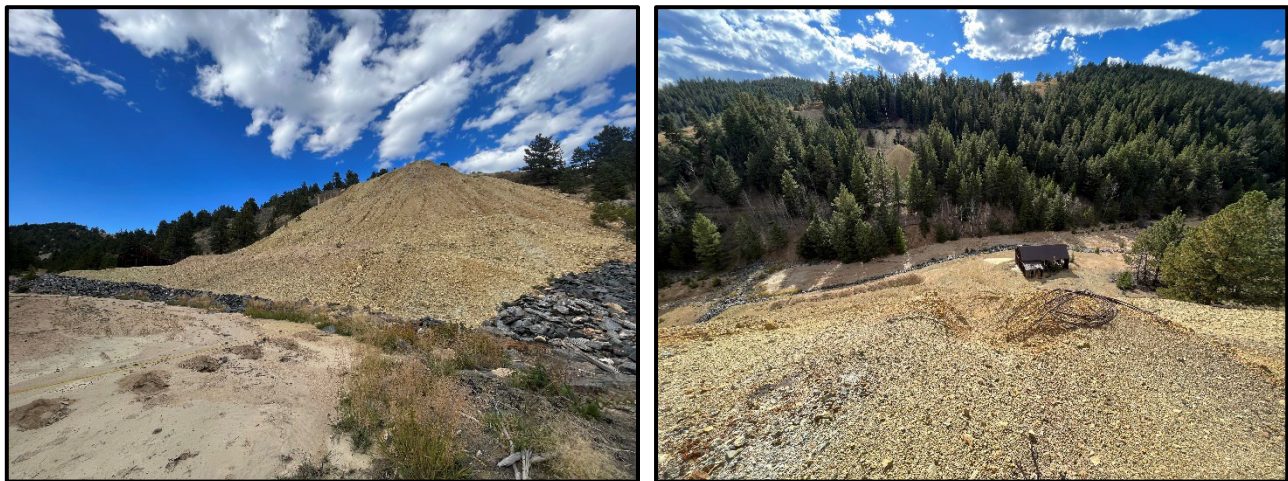
Figure 27. Site #158 – The southeast corner of the previous riprap stabilization work (left) and a downslope view of the southwest-facing slope of the waste pile with Russell Gulch and a historic mine structure at the base (right).
