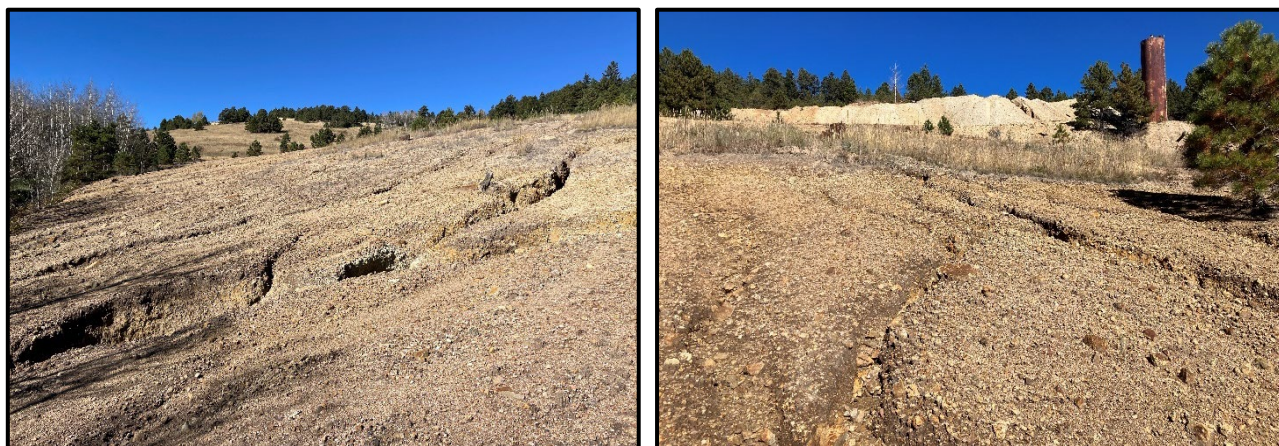
Figure 10. Site #136 - Rill erosion and gully erosion along the toe of the waste pile, looking upslope from left to right.
