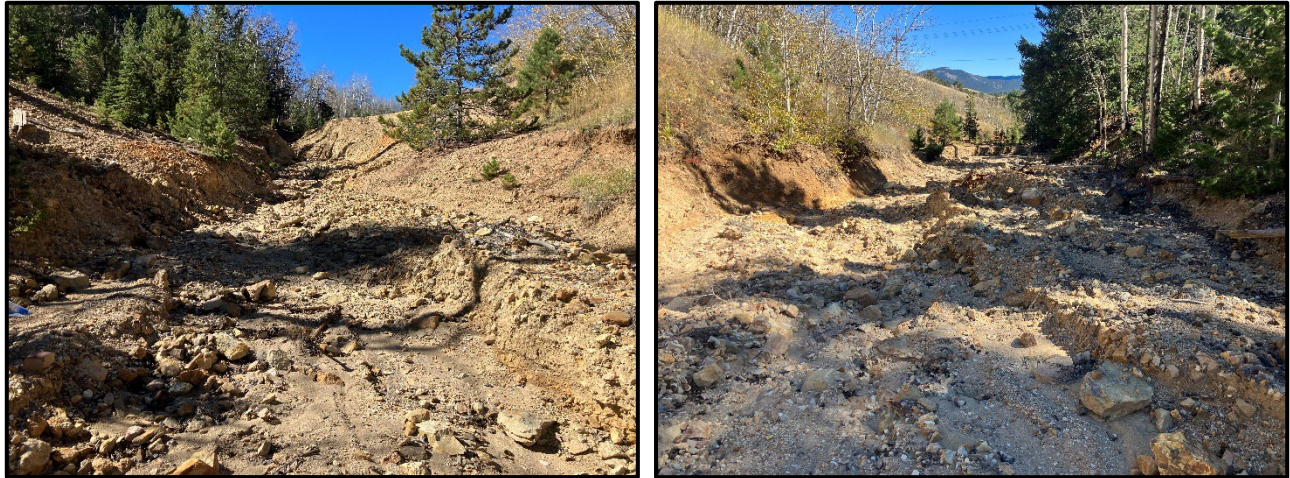
Figure 12. Site #136 - Willis Gulch sediment sample (136-WGDS-SED) location downstream of the waste pile, looking upstream (left) and downstream (right).
