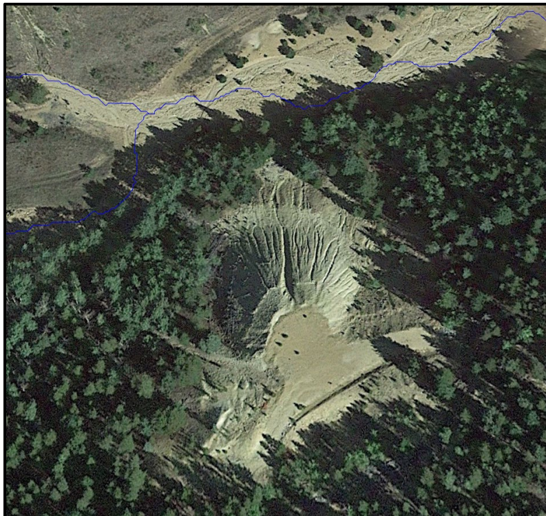
Figure 13. Satellite imagery of the Site #204 waste pile (with numerous rills and gullies) adjacent to Willis Gulch and the South Willis Gulch confluence.
