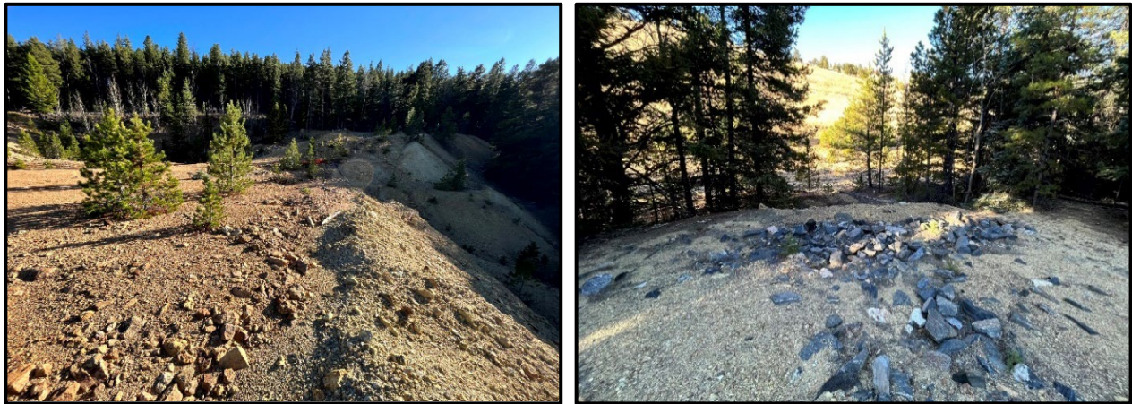
Figure 16. Site #204 – Looking southwest from the top of the waste pile (left) and the toe of the waste pile where sediment has breached a previously installed erosion control feature (right).
