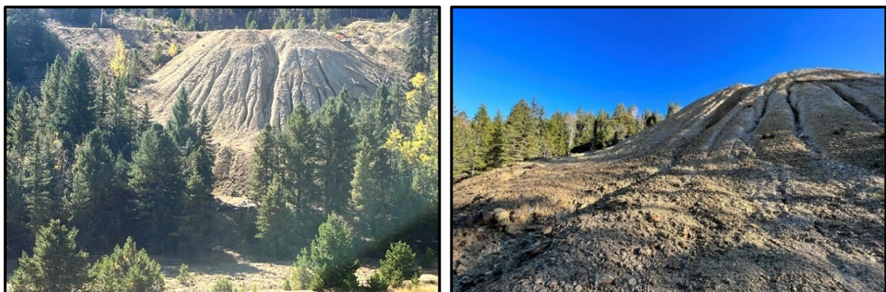
Figure 15. Site #204 - Looking south across Willis Gulch at the waste pile, with a view of the connectivity to Willis Gulch through the trees (left) and the northwest-facing slope of the waste pile (right).
