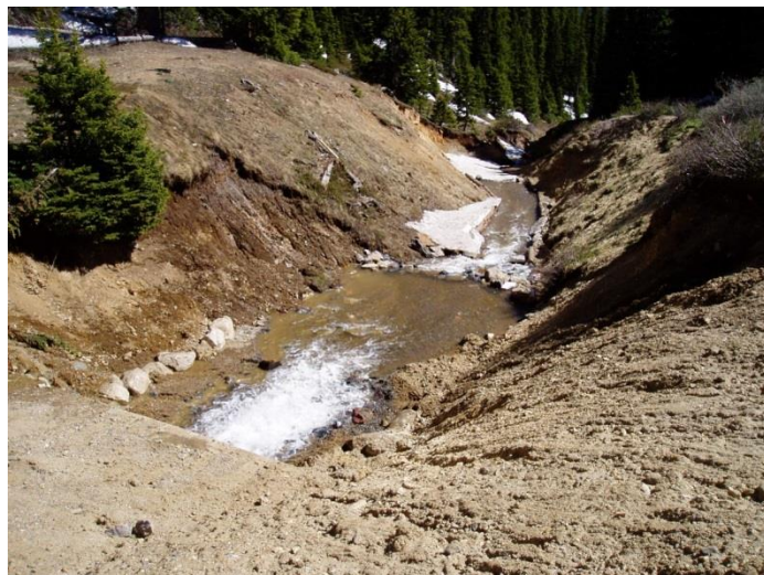
Figure 4-8: Berthoud Pass Diversion channel during construction June 17, 2005
