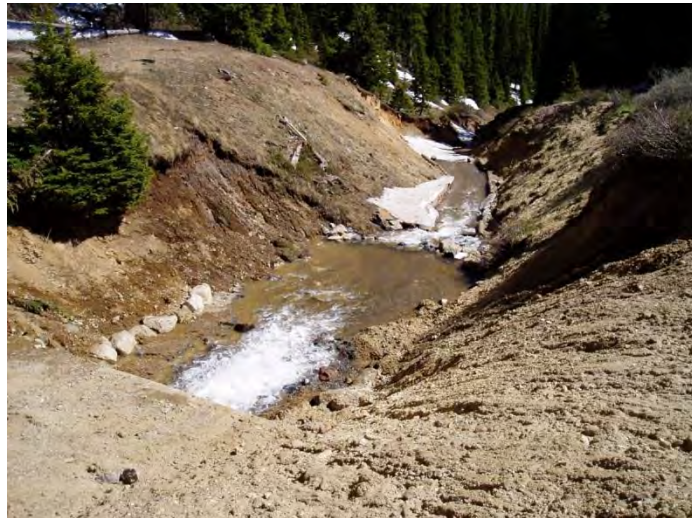
Figure 4-8: Berthoud Pass Diversion channel during construction June 17, 2005
