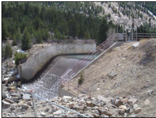
Georgetown Dam Spillway, which Feeds Directly into Clear Creek
