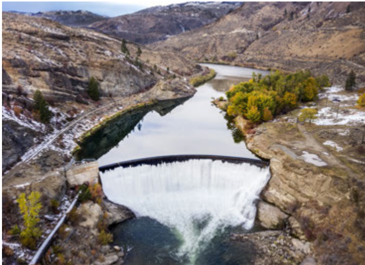
Figure 4.5 Example of Existing Concrete Human-Made Dam [11]
