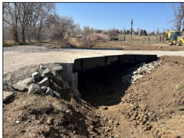
Private driveway crossing with riprap
