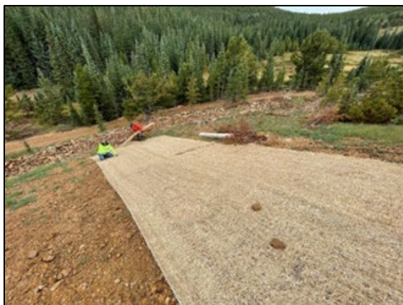
Snowden Mine: Contractors laying erosion control matting across reseeded slopes.
