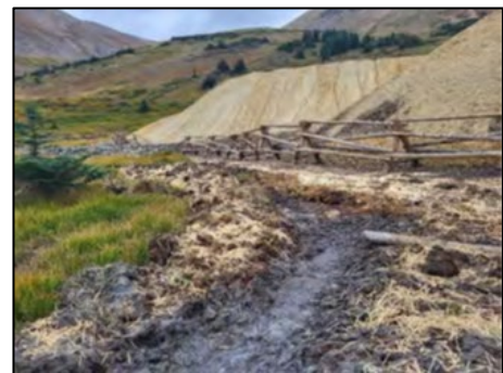
Waldorf Mine: newly constructed containment channel
