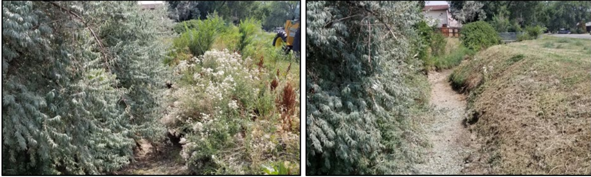
The Church Ditch before (left) and after (right) vegetation removal
