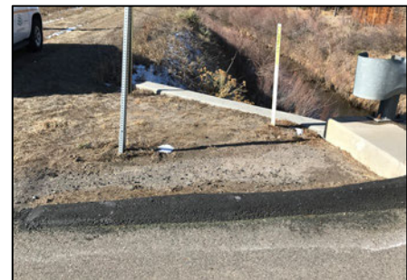
Berms Installed by the City of Arvada
