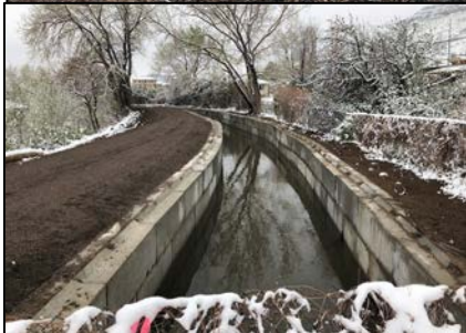
Church Ditch – Area 15 lining before (top) and after (bottom)
