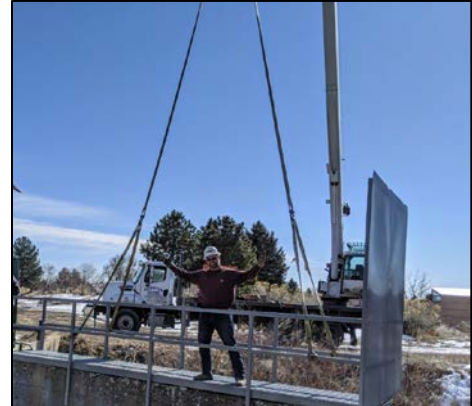
Installation of the new walkway
