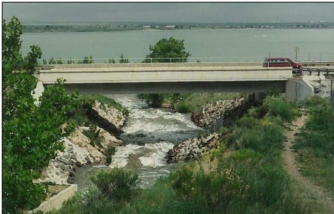
Site where the FHL and Croke Canal enter Standley Lake
