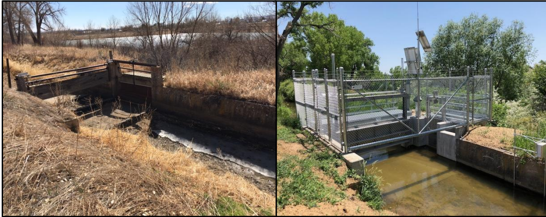
Figure 4. Leyden Flush Structure Before (left) and After (right) Improvements
