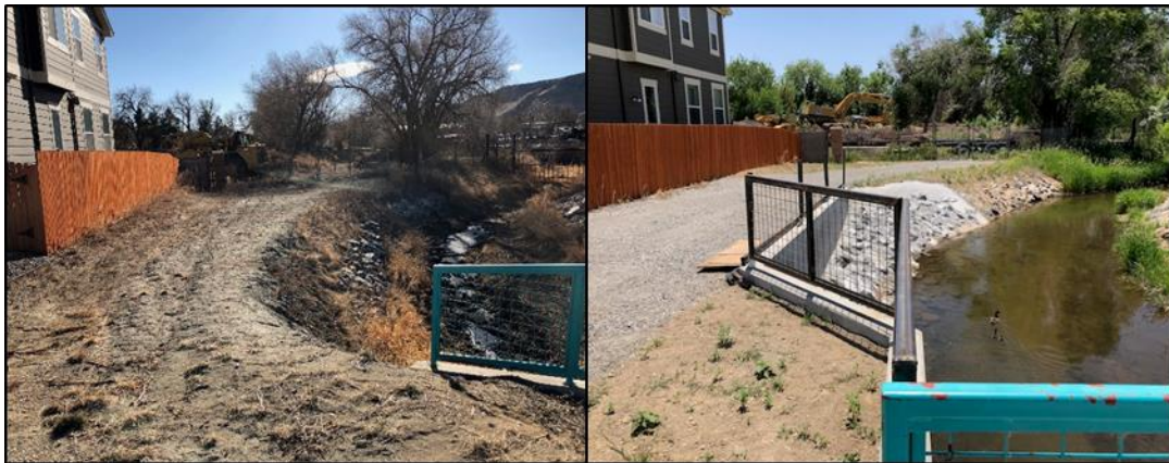
Figure 5. Church Ditch Easement Before (left) and After (right) Improvements
