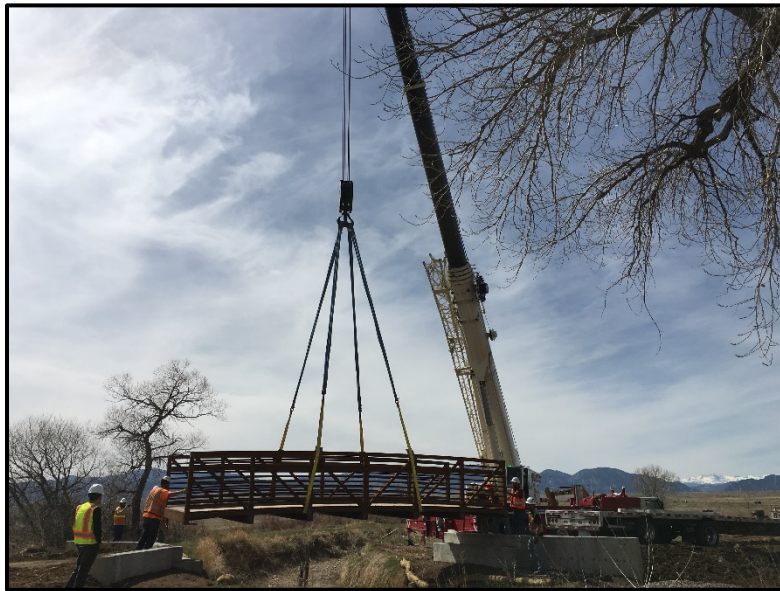
Installation of new pedestrian bridge over Church ditch
