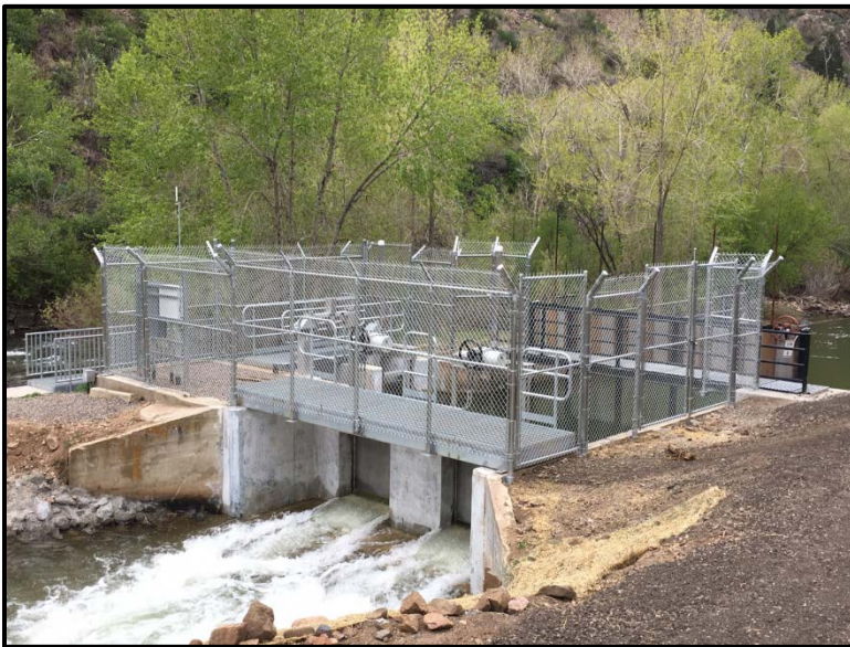
New Church ditch headworks structure.
