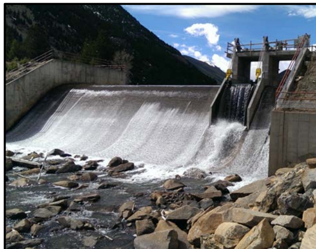
Georgetown Dam, with New Eight-foot Outlet Gate in Operation
