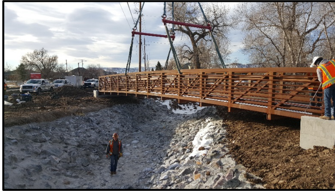
Installation of Bridge Over FHL
