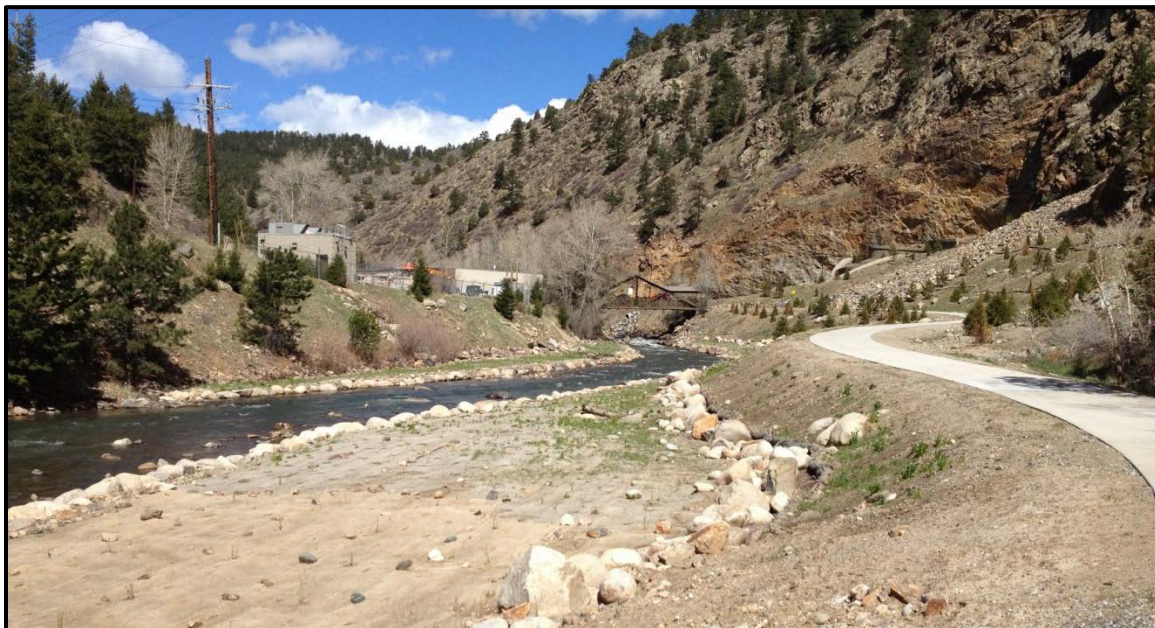
Clear Creek Channel After Twin Tunnels Project, Demonstrating Increased Sinuosity and Expanded Floodplain (Photo Credit: CDOT)
