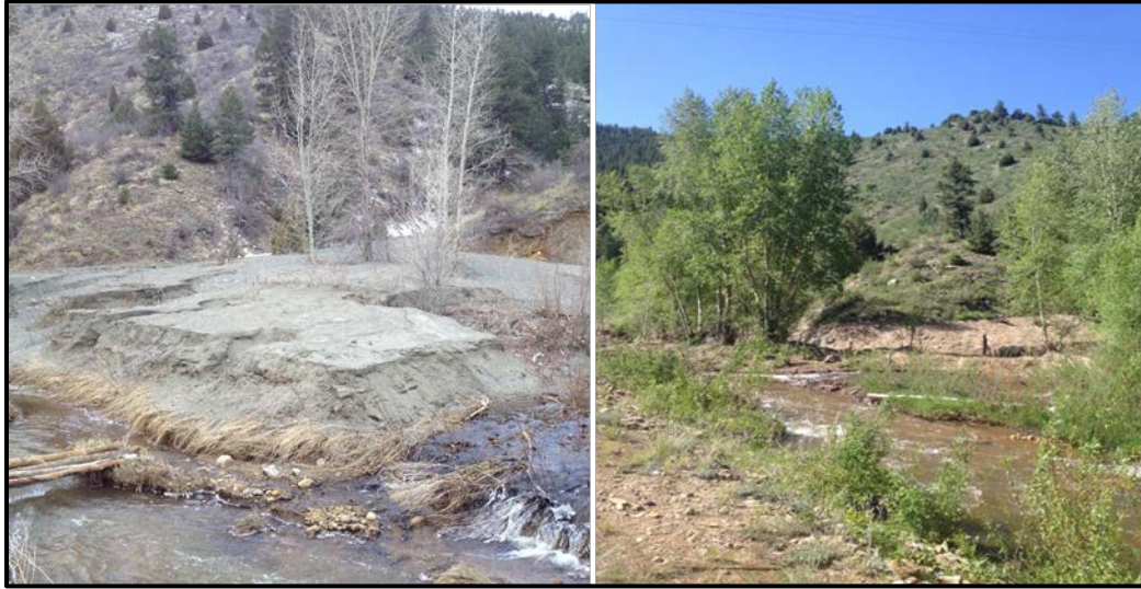
North Fork of Clear Creek Sediment Removal. Sediment Fan after the September 2013 flood (Left). Same location following the remediation and removal (Right). (Photo Credit: CCWF)
