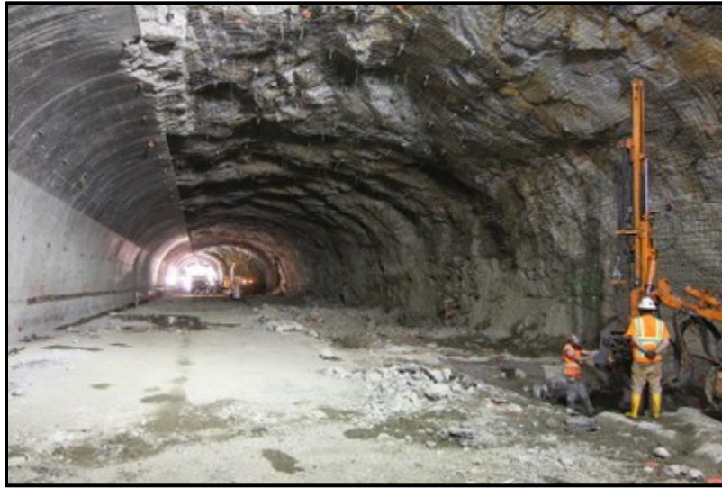
Inside the West-bound Twin Tunnel Bore (Photo Credit: CDOT)
