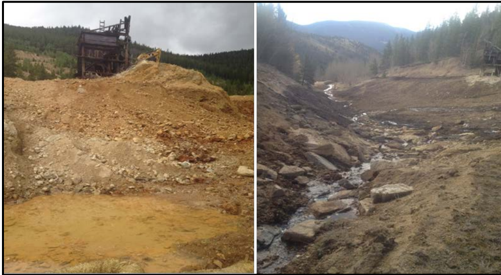
North Empire Stream Corridor Restoration. Ore bin of the Conqueror mine atop an 18,250 CY waste pile within North Empire Creek (Left). Final grade in Upper North Empire Creek after removal of the Conqueror mine waste pile (Right). (Photo Credit: CCWF)
