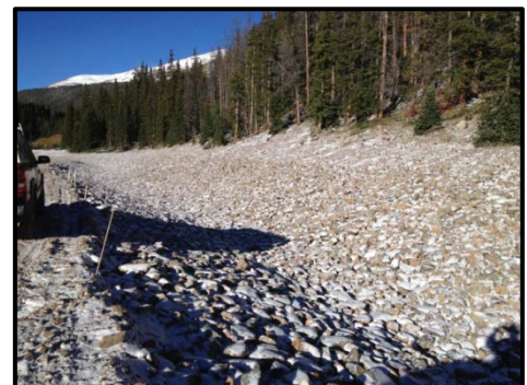
Upper URAD Channel after Construction. (Photo Credit: Freeport-McMoRan)
