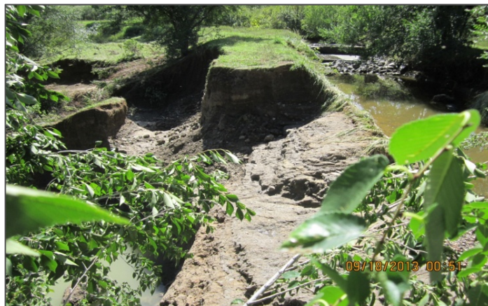
Figure 11. Extensive Bank Erosion on Church Ditch by Leyden Creek after the September 2013 Flood Event (right)
