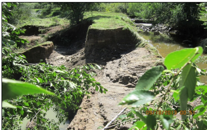
Figure ES-2. Extensive Bank Erosion on Church Ditch by Leyden Creek after the September 2013 Flood Event (right)
