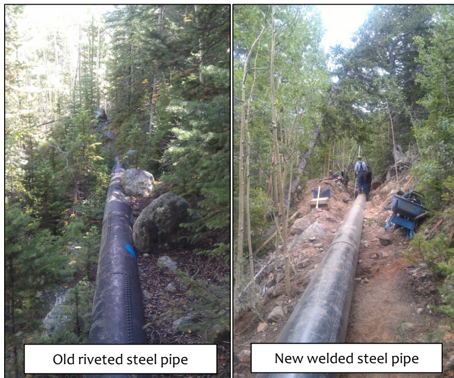
Figure 25. New section of pipe from Leavenworth Creek toward Green Lake
