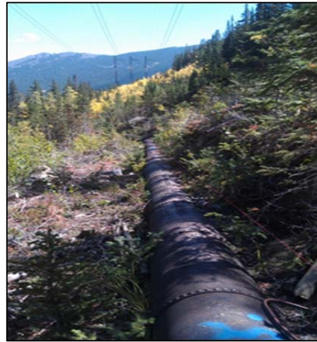
Figure 22. New Pipe from Leavenworth Creek toward Green Lake
