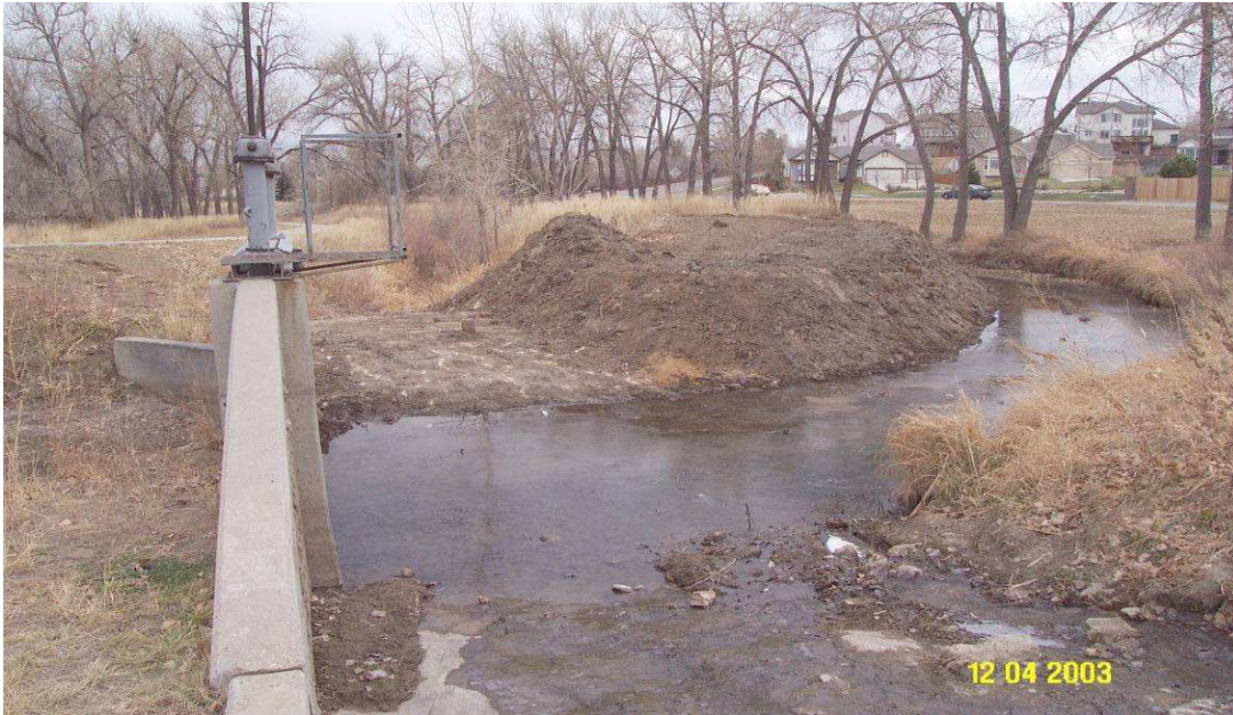
Figure 26. Old ditch structure. Ditch in center of the photo with Little Dry Creek inflows on bottom right.
